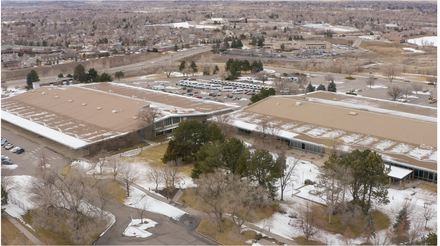
Lightning eMotors expands into a second building (on the right)
